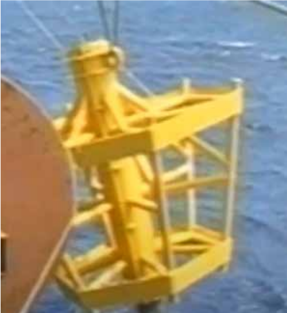
Fig.5.7: Picture of WSW intake segment (Installation)
