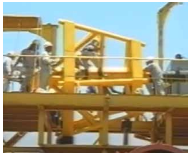
Fig.5.6: Picture of WSW intake segment (Assembled in the construction)
